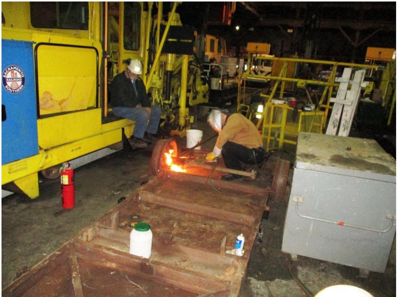
Alan watches as Kyle torches the axel connection points on the wide-treaded wheel flatcar
