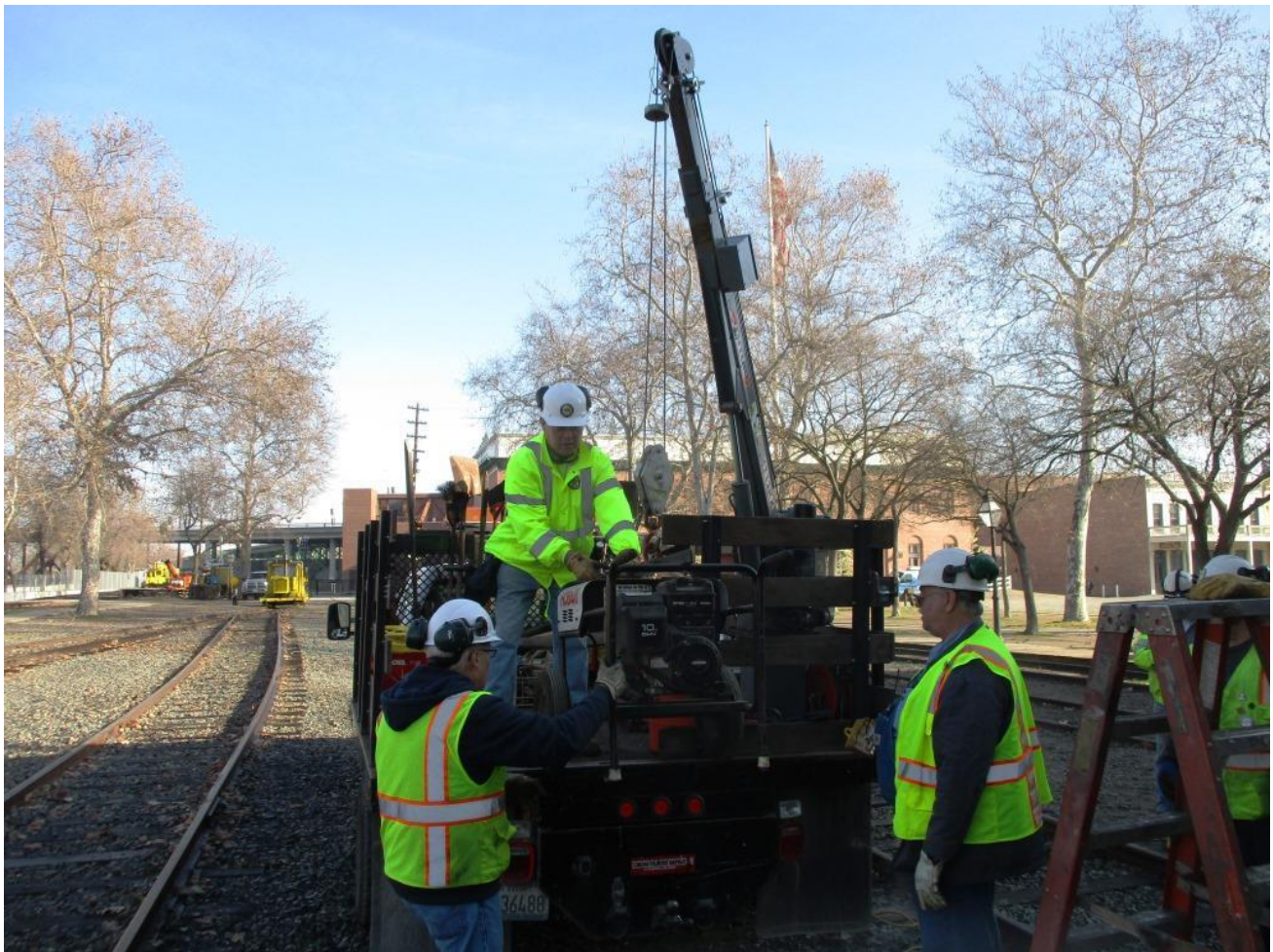
Taka, Bill, and Chris C. use the truck's crane to deploy the portable welding unit
