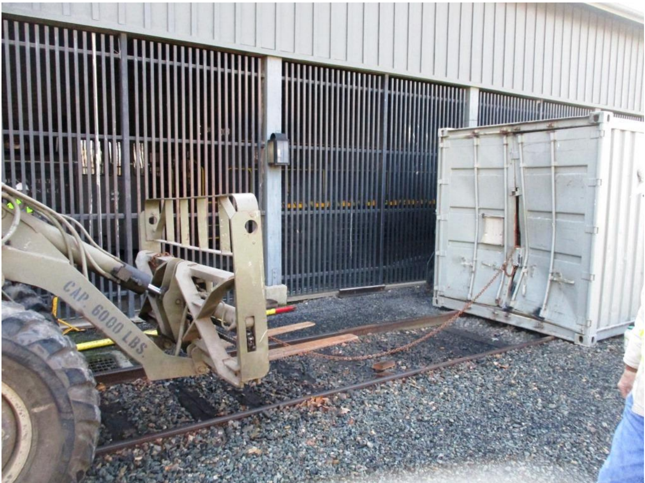
With the rods now separated from their latches, a chain is hooked up between the container door and GM2...
