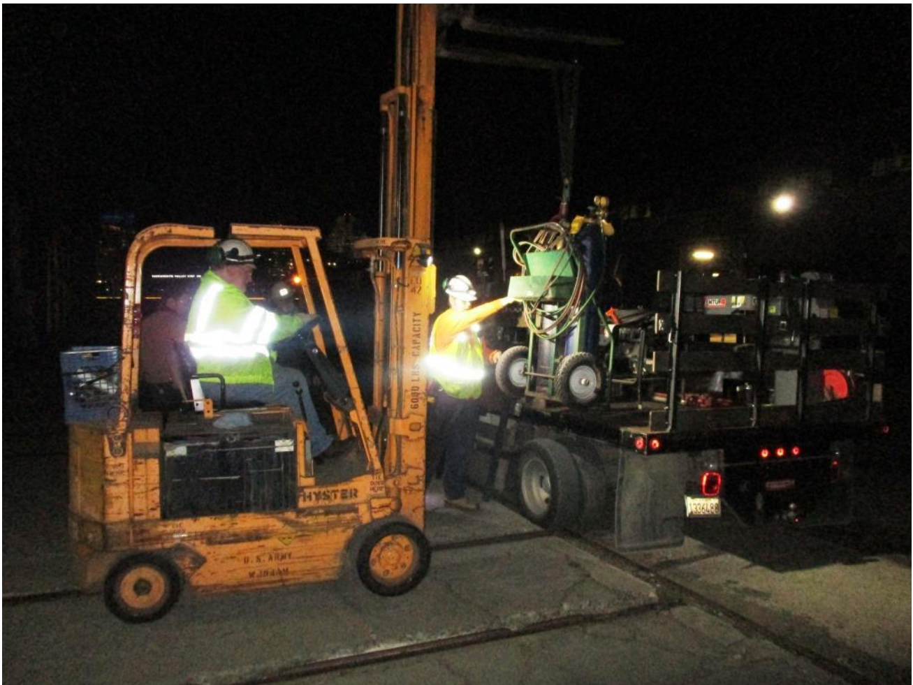
Frank, on the forklift, loads the oxy-acetylene tanks on the truck with Chris H. as guide
