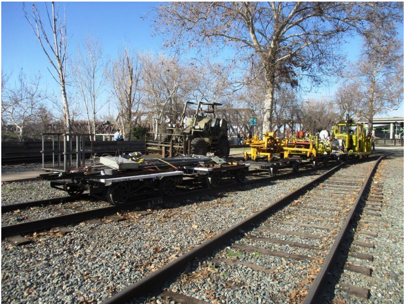
The flatcars containing the rail and conduit along with the damaged equipment are shuttled back to the Shops
