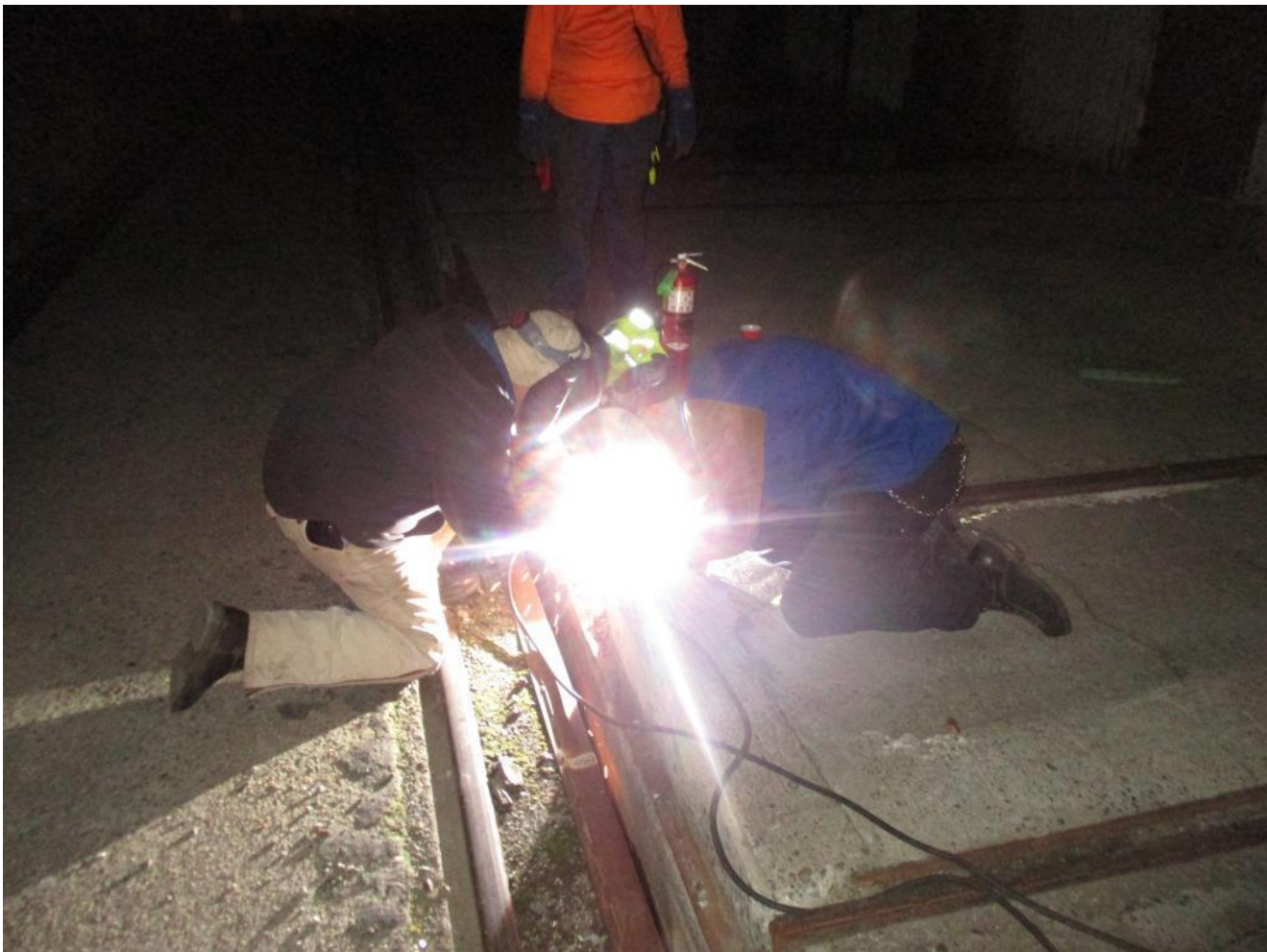
Cliff and Kyle weld the busted rail-ramp into place at Track 5 on the transfer table apron
