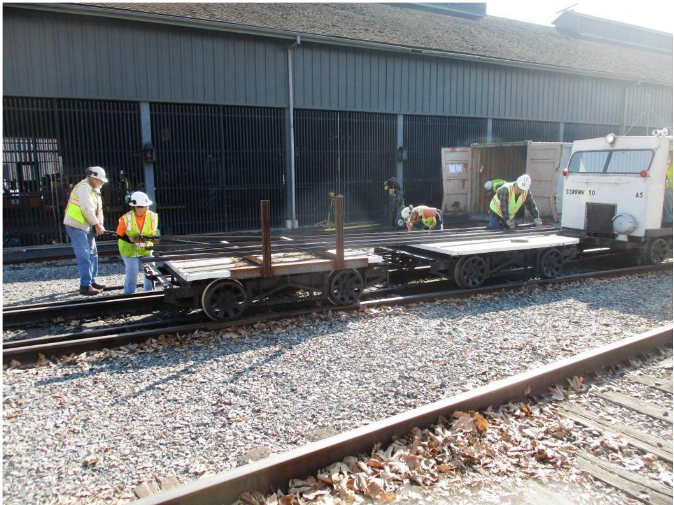
Alan, Pam, Mike F., and John load the rails removed from inside the container on flatcars
