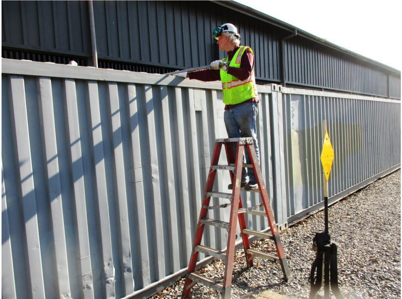
Steve removes a bracket holding the electrical mast from the roof of the container
