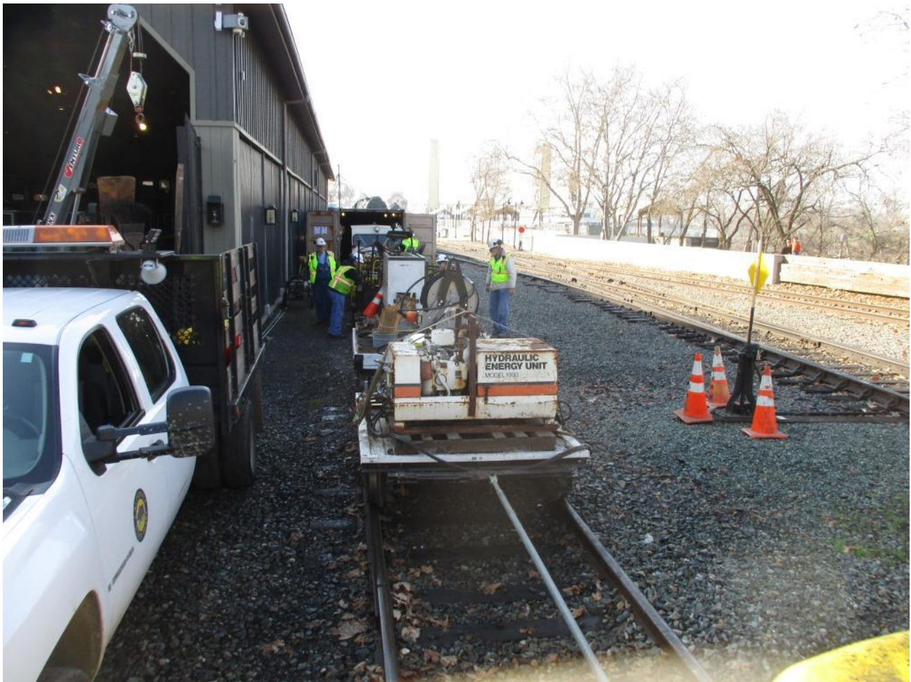
With everything out now, a damage assessment is undertaken
