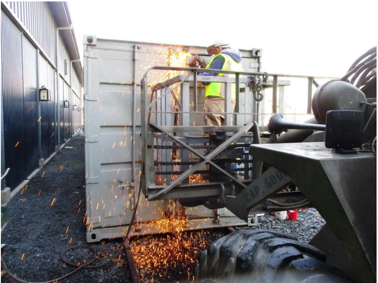
As Cliff separates the locking bars from the latching cleats, great "BANGS," like gun-fire were heard as tension is released on the rods
