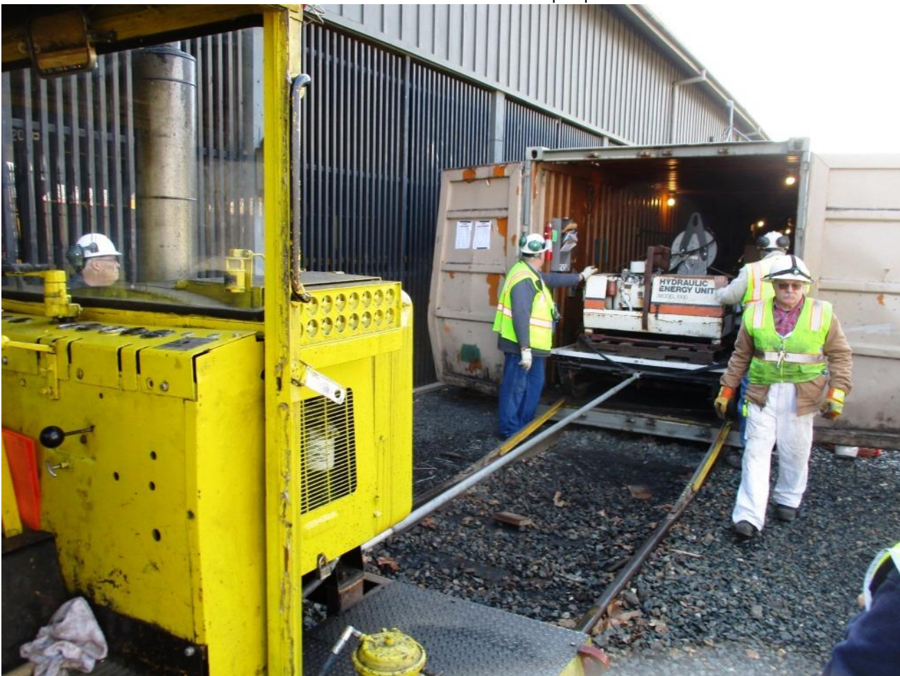
The Kalamazoo is brought in and, using a long drawbar, the equipment is extracted carefully from the container
