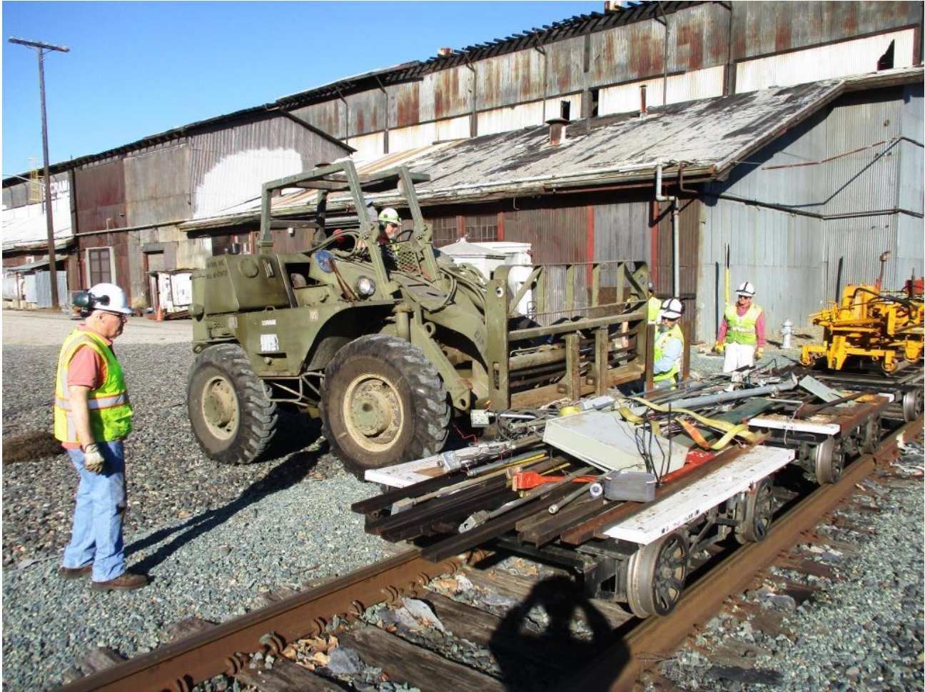
Bill, Joe, and Mike H. work with Mike F. on GM2 to remove materials from the flatcars
