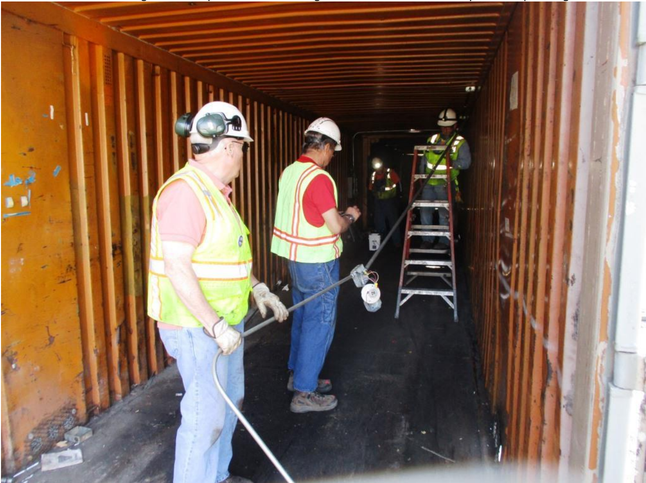
Bill, John, and Joe remove conduit from the ceiling of the container
